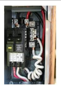
Customer must provide pigtail with wires inside conduit from subpanel to spa base, pigtail MUST be a minimum of 4' from base of tub in order to make final connection. We will cut off excess wires in making final connection. IF WIRES ARE NOT INSTALLED PRIOR TO DELIVERY WE WILL NOT BE ABLE TO START YOUR SPA ON **DELIVERY.**
