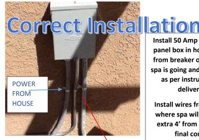
**Install 50 Amp Breaker in main** panel box in house. Run wires from breaker out to where the spa is going and install subpanel as per instructions in predelivery guide.
